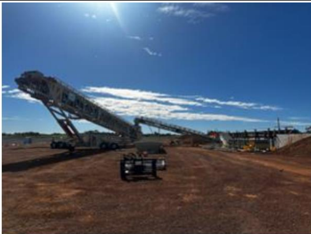
Figure 6: Ruvidini Inland Port construction – July 2024
